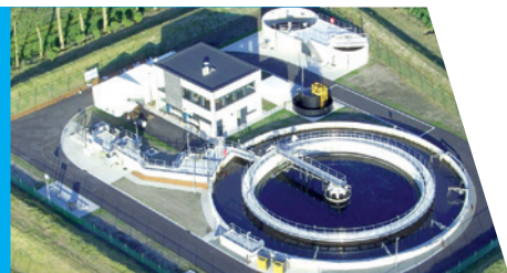
Small scale wastewater treatment plant in Belgium (Photo: Aquafin)
