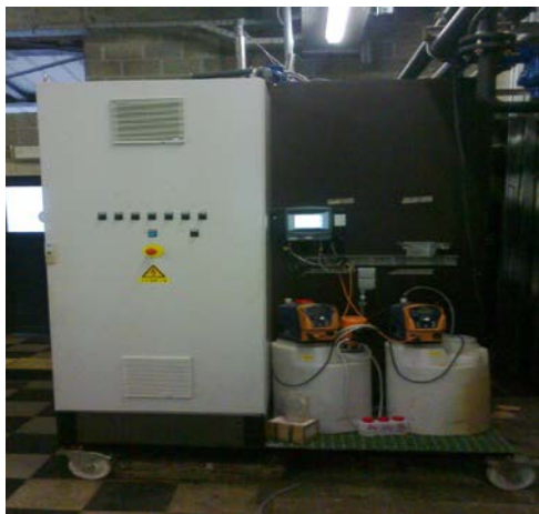
Anammox pilot scale reactor (Leuven WWTP, Belgium)
