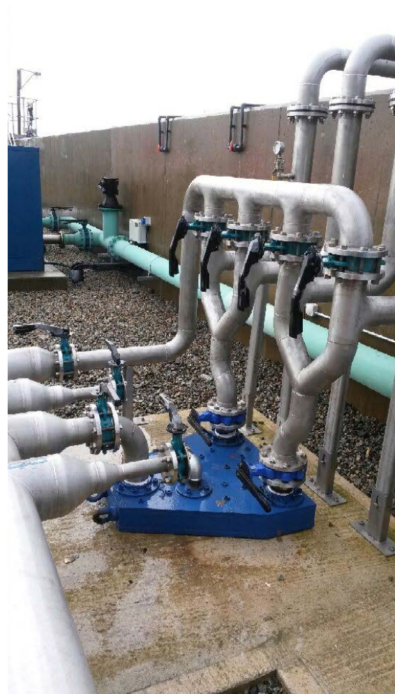
DN100 Oscillator in operation at a facility in the Republic of Ireland.
