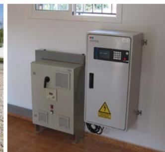
The OptimEDAR solution is composed of a control cabinet and a sensors cabinet installed in the bioreactor. Data transfer between cabinets is done by wireless connections, simplifying installation and reducing their costs. In addition, it includes a GPRS/3G connection and a data collection software is delivered in order to manage and monitor the system.
