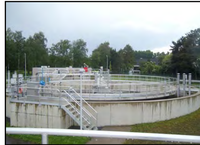
Wijer WWTP (1.600 P.E., Aquafin)
