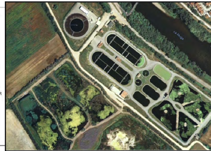
Empuriabrava WWTP (70.000 P.E. CCB)
